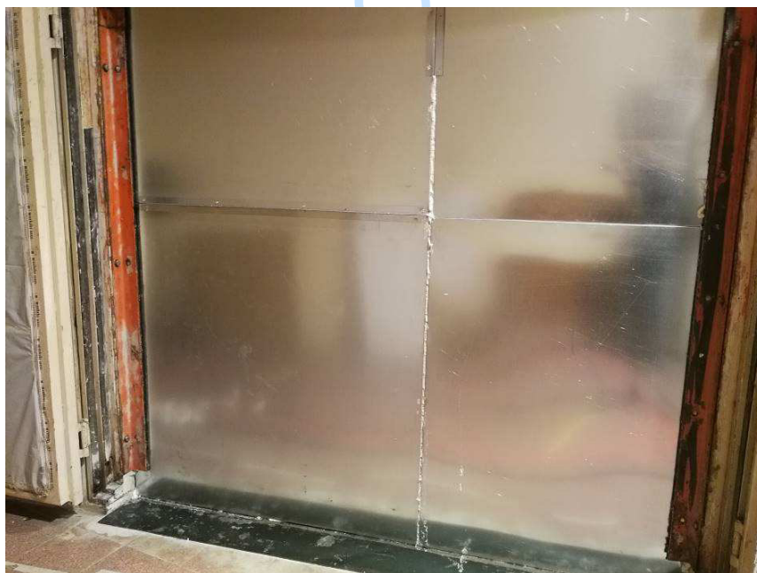
Lato camera ricevente / Receiver room side
